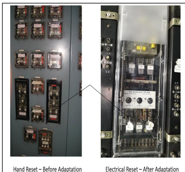
Figure 6. Adaptation of Relays for Remote Reset
