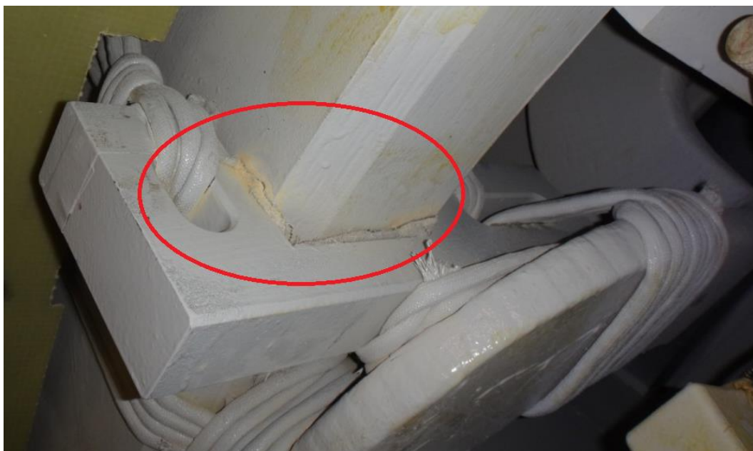
Figure 4 – Loose blocking near 11:00 Jumper Connection in 2015
