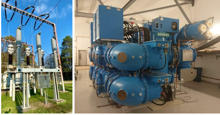
Figure 9 Sensgear installations for a CO 2 neutral / blue Circuit Breaker (left) [7] and a blue GIS (right) [8]
